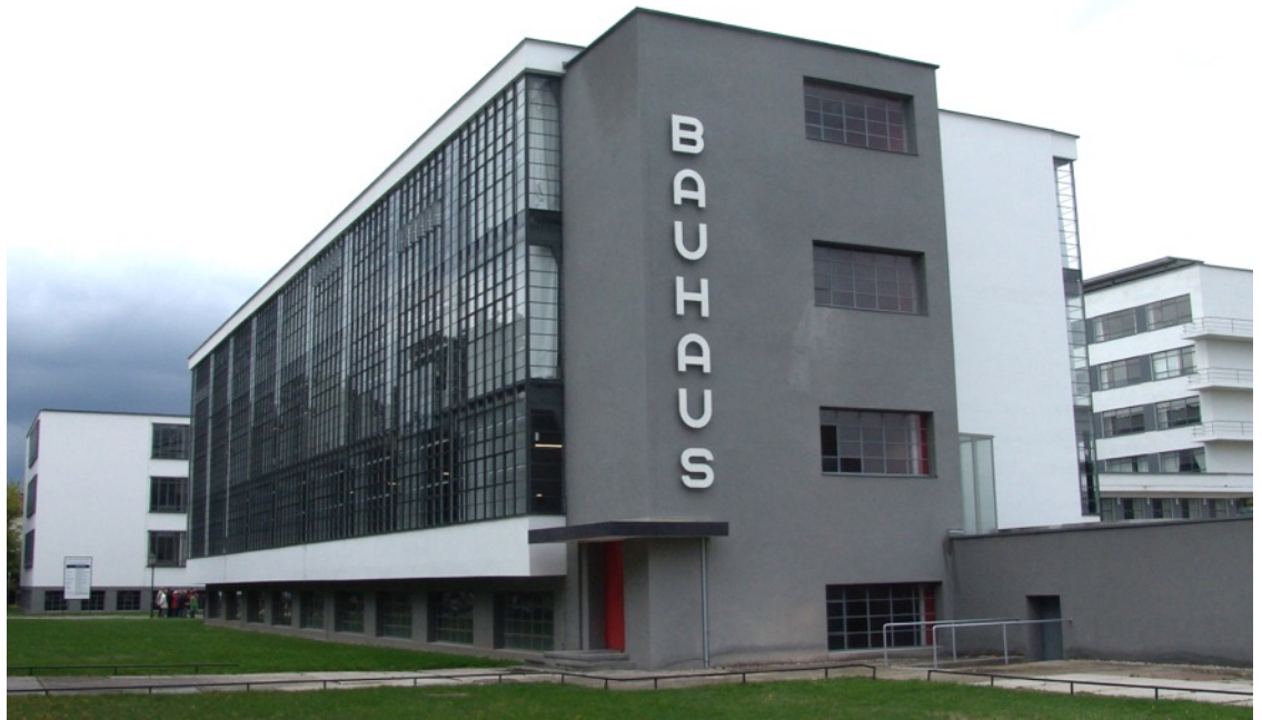
Bauhaus in Dessau, Germany (2005) Architect: Walter Gropius
